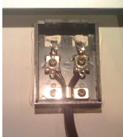
Figure 2. Solar Panel Wire Connection
